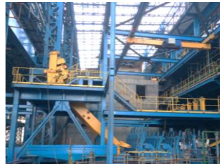
Steel Structure for WSU Unit
