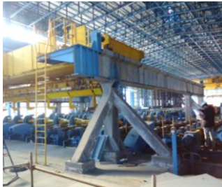
Support Structure for Cross Transfer Area
